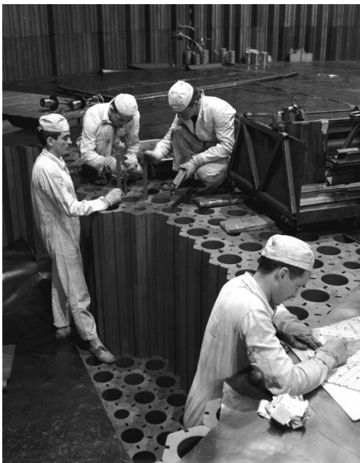
Figure 1: Chinon A3 Core Assembly in 1965 (EDF Mediatheque / Brigaud Michel)
